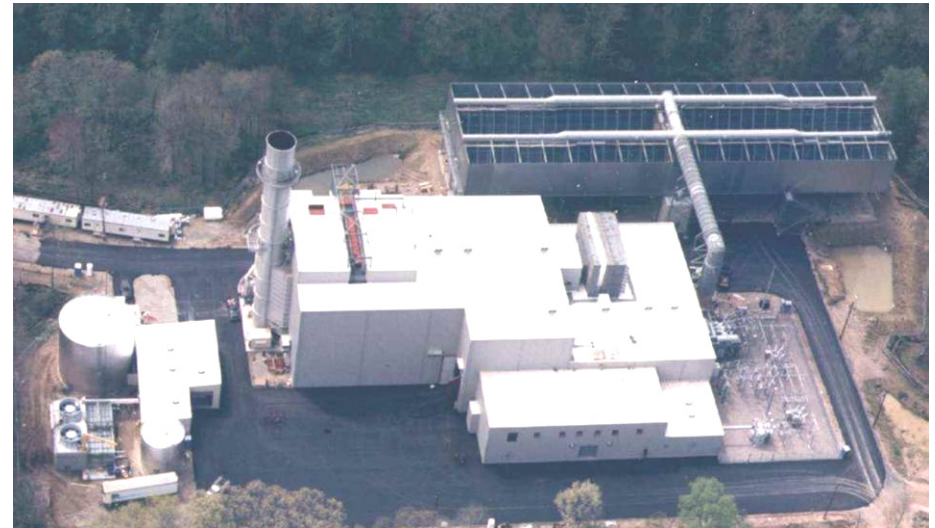
Gas Turbine – Over 34,000 MW
