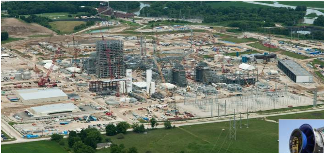
Edwardsport IGCC project, USA
